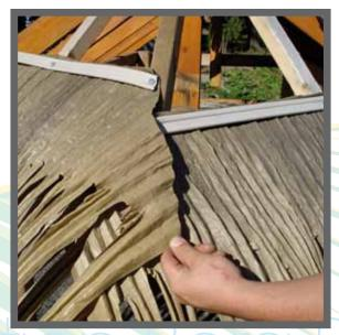
1) Firstly, cut the edge of the leaf at the junction to get a clean corner angle, cutting from the top rail **following** along the beam and up to the start of the next row (the one just below). THEN, from that point cut at a 60° angle. Fix the rail to the beam.
