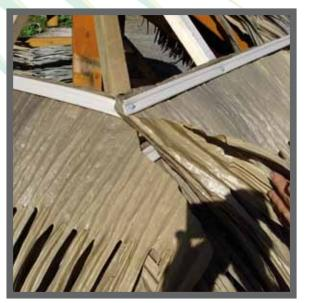
2) For the other side of the same junction, cut at a 60° angle starting from the top of the rail to the end of the leaf. Fix the rail to the beam.
