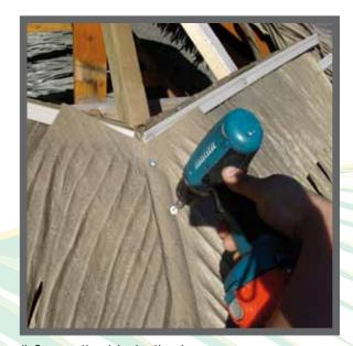
3) Lay a hip at the center of the vertical beam, starting at the rail. Screw the hip to the beam (minimum two screws).
